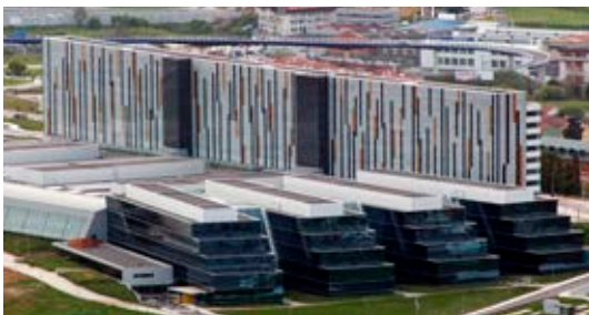
Huca Hospital, Asturias Spain is one of the country's most significant hospitals covering nearly 190,000m 2 .
