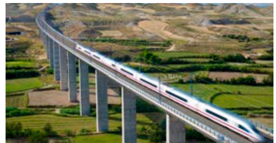
Spain has the second longest high speed rail network in the world. TMC is a homologated supplier to ADIF, the network manager and has supplied a significant portfolio of transformers across various applications.
