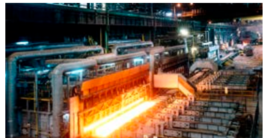
ArcelorMittal steel plant in Asturias, Spain produces 1,2 million tonnes per annum of blast furnace-basic oxygen furnace (BF-BOF).
